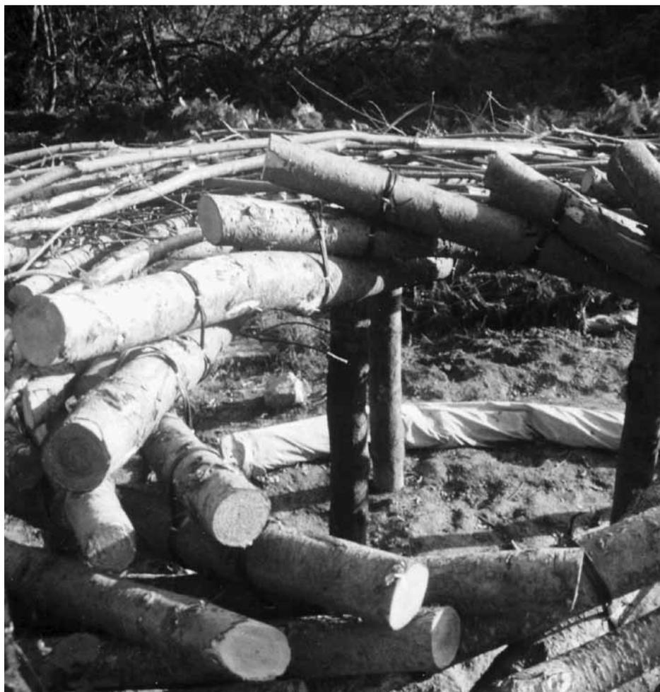
*Detail of telephone wire strapping around the skylight hole.*
