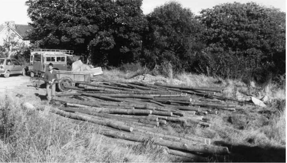
*This is the amount of wood needed for the structural framework.*
